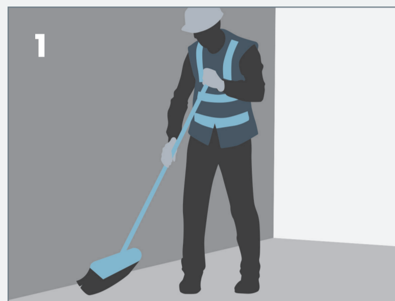
1 Ensure the substrate is clean and dry.
